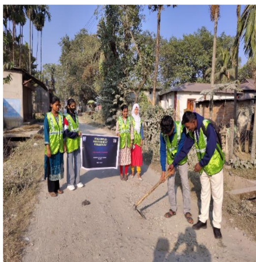
Road repairment programme at subhaspally by NSS unit II volunteers
