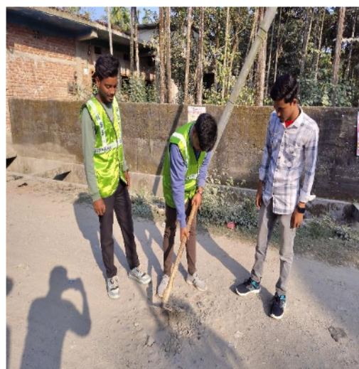
Road repairment programme at subhaspally by NSS unit II volunteers
